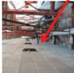
Crossing point for brace to be used as a top rail must be 38" to 48" above platform.
