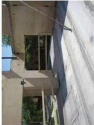
Must be erected to protect the worker along each unprotected side or edge. They also must meet very specific height and strength requirements. Workers erecting the rails must be protected while doing so.
