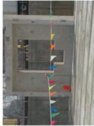
A barrier used to warn workers of an unprotected side or edge. Also used to designate the area where work activities are taking place under an alternative fall protection plan.
