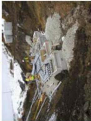
Sloping at a safe angle (based on soil type) prevents or minimizes the risk from a collapse.
