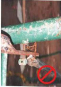
Cross braces, horizontal braces, diagonal braces, or a combination of braces must be used to secure vertical members to prevent collapse.
