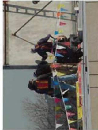
Must be used as part of a complete fall protection plan and only in certain instances such as leading edge work, precast concrete erection, some roofing work and residential construction work.
