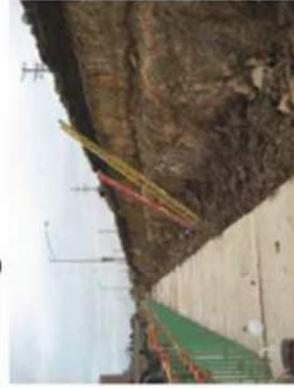
Benching requires the same overall angle as sloping. This technique can be used only in soil types A and B.
