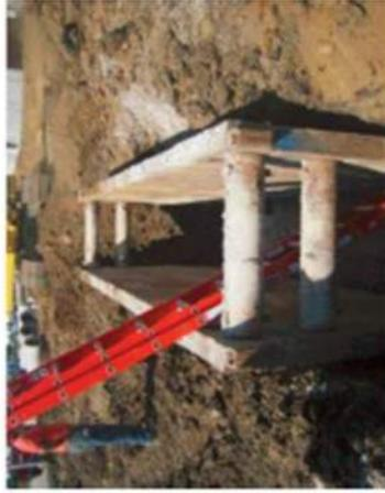
**Spoil Piles:** All soil and rock removed must be piled back at least 2' from the excavation to help prevent collapse and falling objects.
